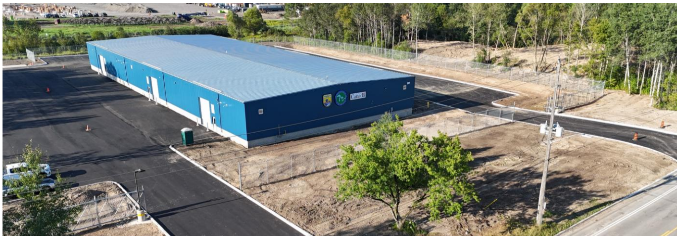
Photo of the completed Commission facility. (Rand Construction)
